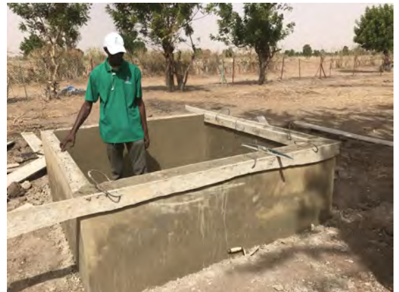
Lead Contractor Abdoulaye Kane surveying the work
