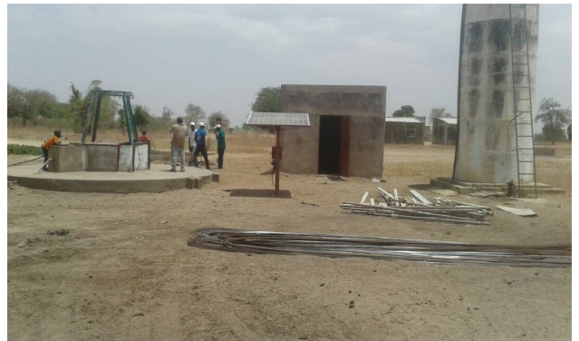
Crews installing the pump & tank structure
